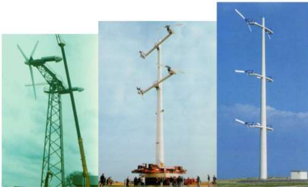
Figure 4: (Left to right) Twinmaster, Quadro [11] and Sixmaster [10] built by Lagerweij Wind
